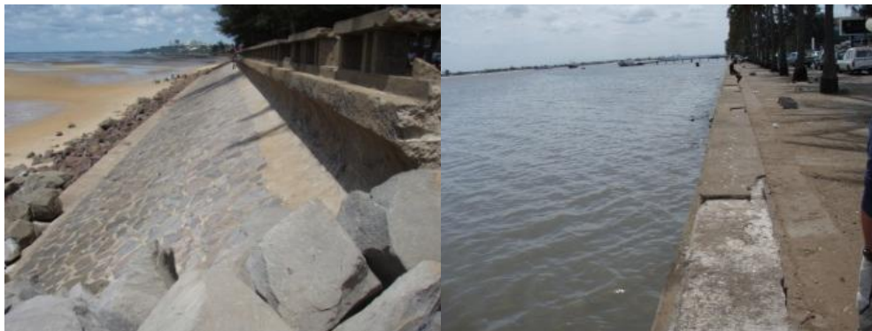
Figure 5: Examples of a revetment (left) and a seawall (right) in Mozambique
