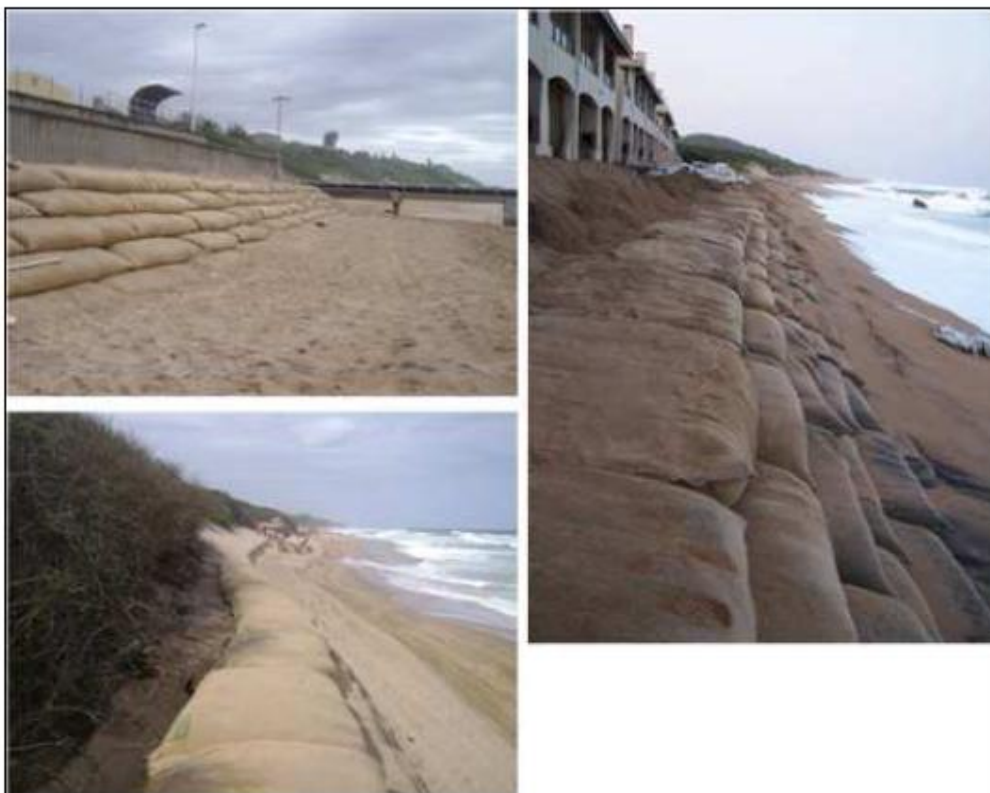
Figure.15: Examples of geotextile (sand bag) revetments (Kwazulu-Natal, South Africa)
