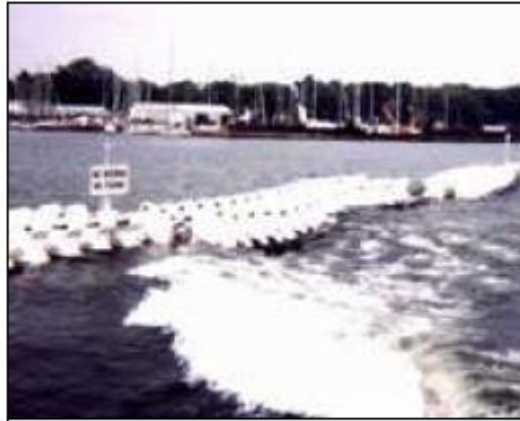
Figure 14: Patented floating breakwater (www.whisprwave.com)
