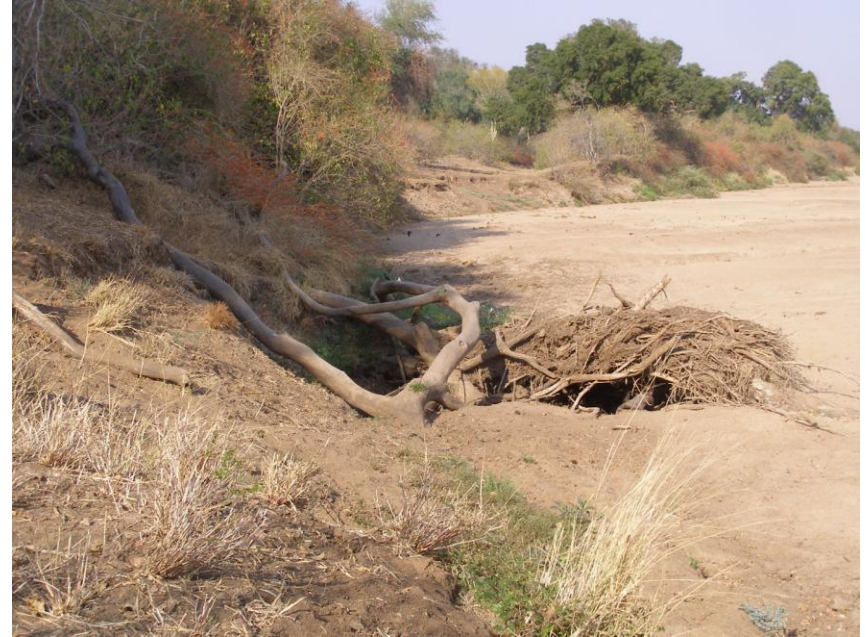
Bank eroded by 2000 flood – Up to 60 m lost
