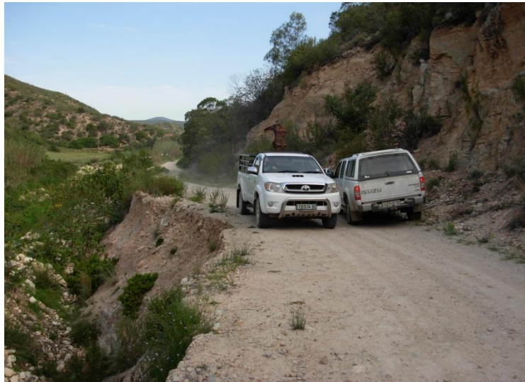
Picture 5. Damage to roads that have not yet been repaired. Photo Source: Author
