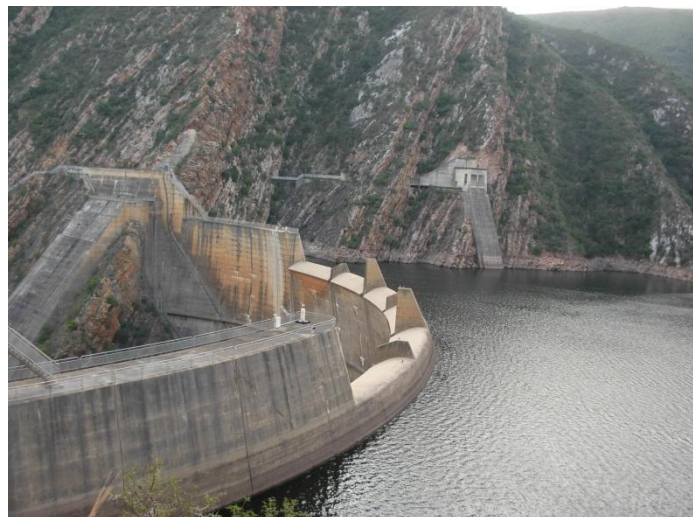
Picture 6. Built in 1969, the Kouga dam stores 129 million m 3 of water and is the key water source for the Nelson Mandela Bay Metropolitan Municipality. Photo Source: Author
