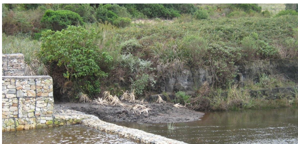
Photo 9: Incised peat wall exposed to desiccation in hydro-geomorphic unit 2
