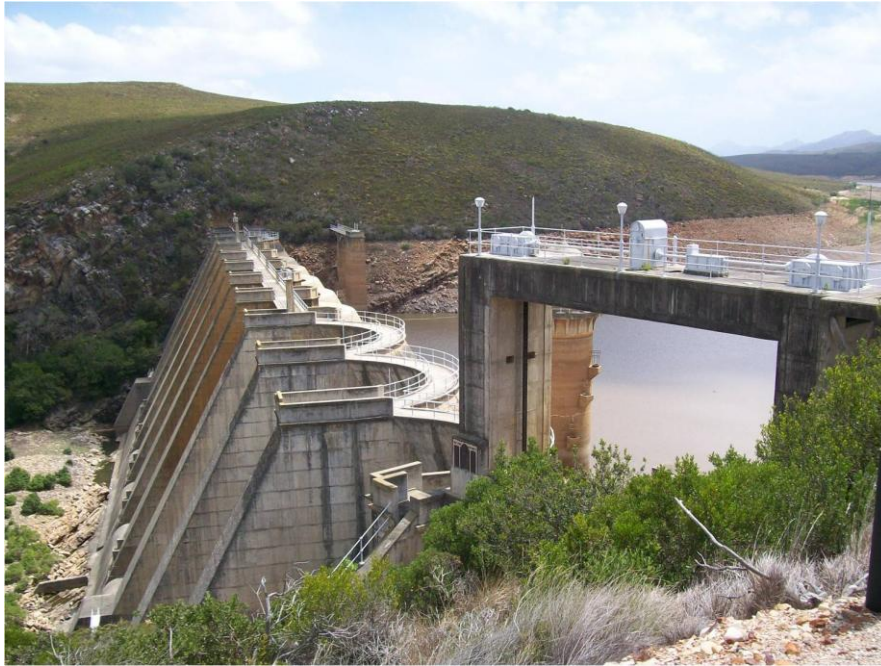
Figure 3.18: The multi-arched Churchill Dam on the Kromme River in the Eastern Cape of South Africa
