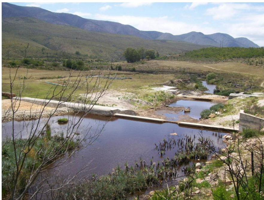
Figure 3.9: Cement weirs built along the Kromme River, Eastern Cape, South Africa. These weirs are built to restore the river by stopping the headcut from proceeding backwards up the river. This traps sediments and allows vegetation, such as P. serratum in this photograph, and eventually wetlands to recover
