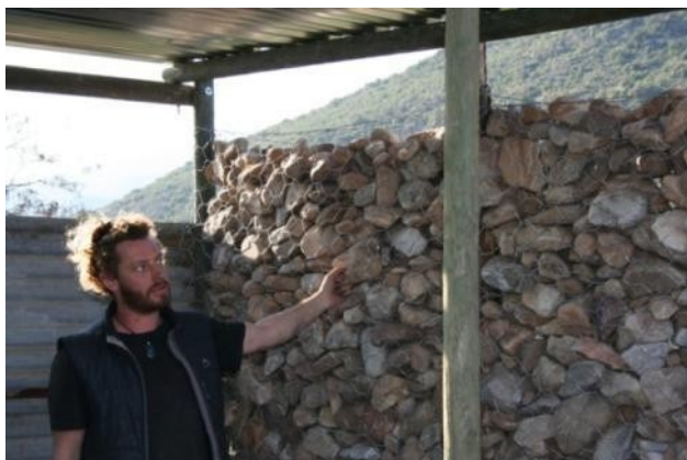
Figure 25: gabion wall
