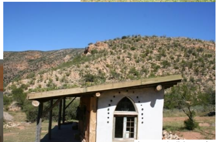
Figure 11: The living roof
